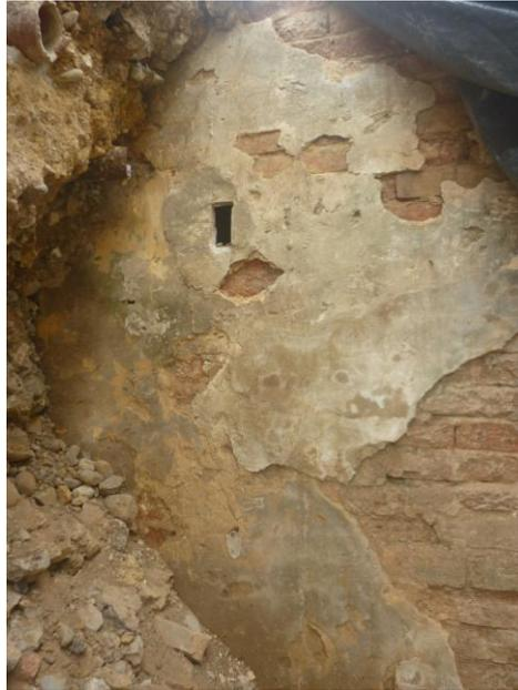
Fig. 4. A sample extraction site of plaster mortar at Puente Ortiz
